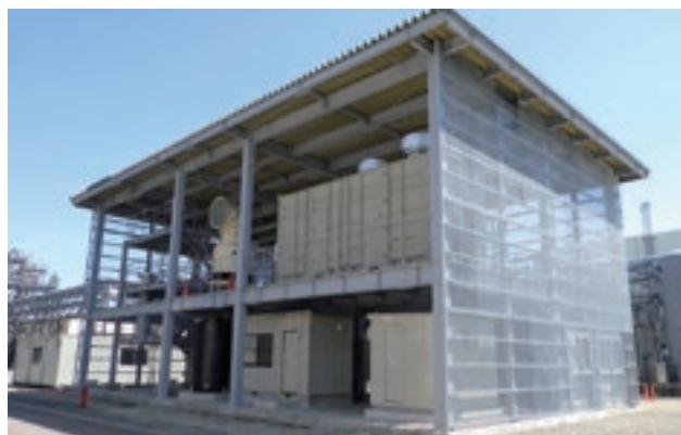
CO 2 methanation test facility currently under construction
