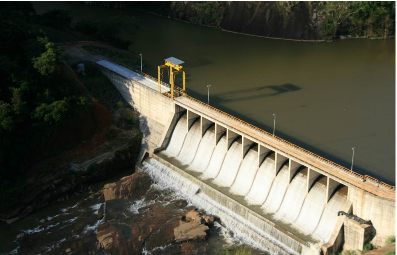
Brazil is a key growth market for Statkraft, and in 2018 a cluster of eight operational hydropower plants was acquired. The hydropower plants are located in the state of Espírito Santo in Brazil, and have a total installed capacity of 131.9 MW.
