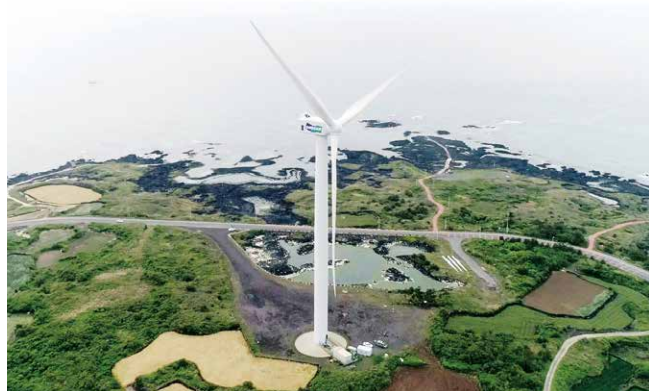
8MW offshore wind power generation system
