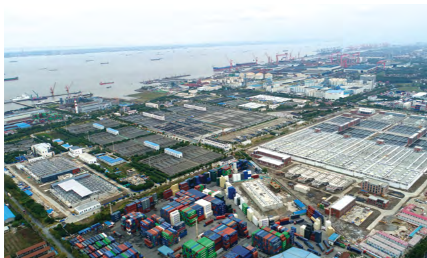
Sewage treatment plants built by SUMEC in Zhuyuan, Shanghai
