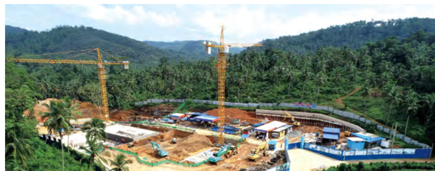
CMEC builds the Astana Water Works in Sri Lanka
