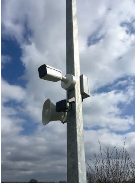
Examples of CCTV with Audio Challenge Installed on Apollo Solar Sites
