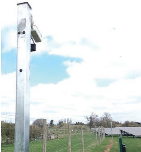
Examples of CCTV with Audio Challenge Installed on Apollo Solar Sites
