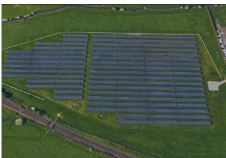
Brook Barn Solar farm
