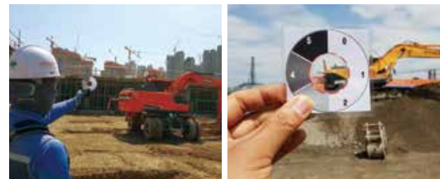
Measuring method for find dust of construction equipment
