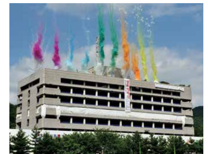
*Explosive demolition at Bundang Office of Korea Gas Corporation (2017. 6. 15)
