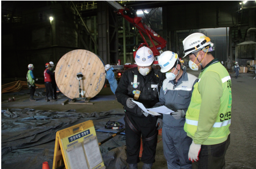
Major repair progress and inspection
