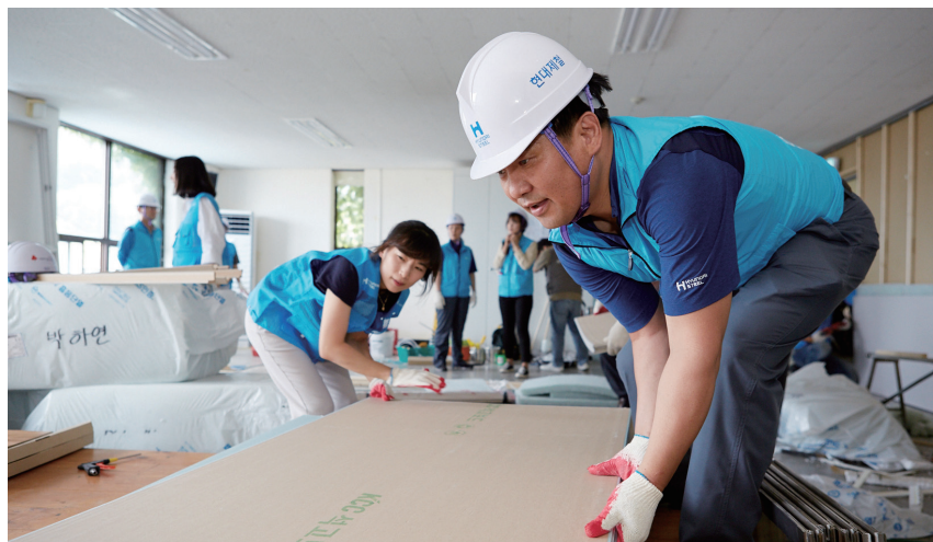
House Repair Energy Efficiency Project of energy efficiency project
