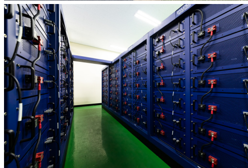
up) FerroPhalt, Eco-Friendly Road Pavement Material down) ESS by recycling EV batteries
