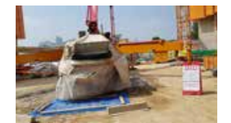
Permit to Work(펌프카 등)
