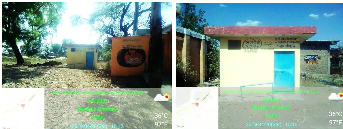
Figure 6: School toilet of Govt. primary school Amlaha, Sehore
