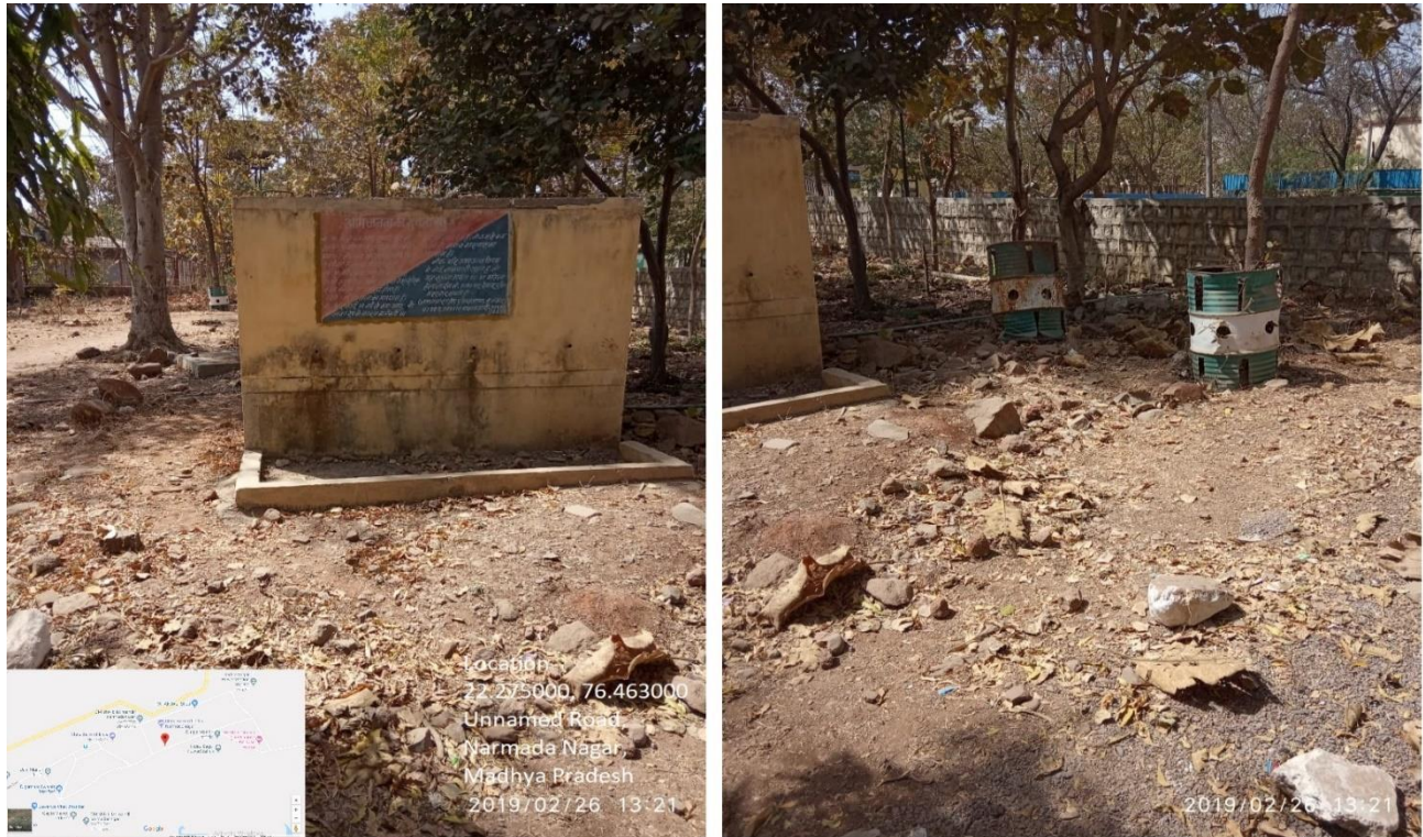
Figure 17 Water Storage Tank with platform in Govt. schools Narmada Nagar
