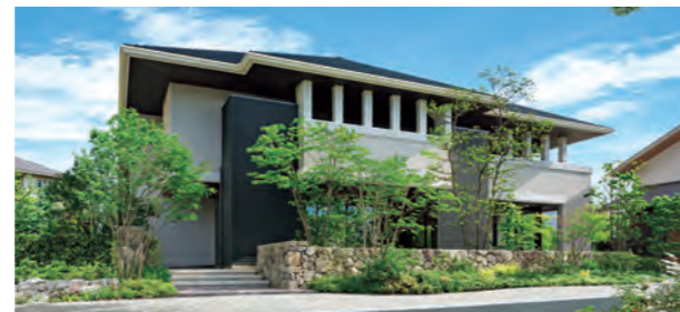
IS ROY+E steel-framed two-story house
