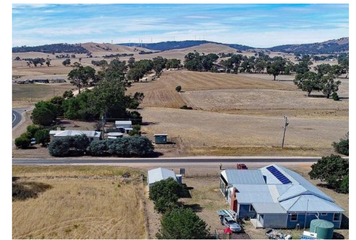
Crowlands Hall rooftop solar installation
