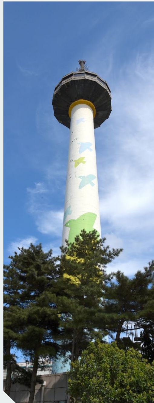
2 — Picture of the Pohang Works Environment Center
