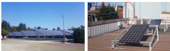
Hyupdong Sports Facility and rooftop of the Electrical Steel Plate Sub-Center No.3
