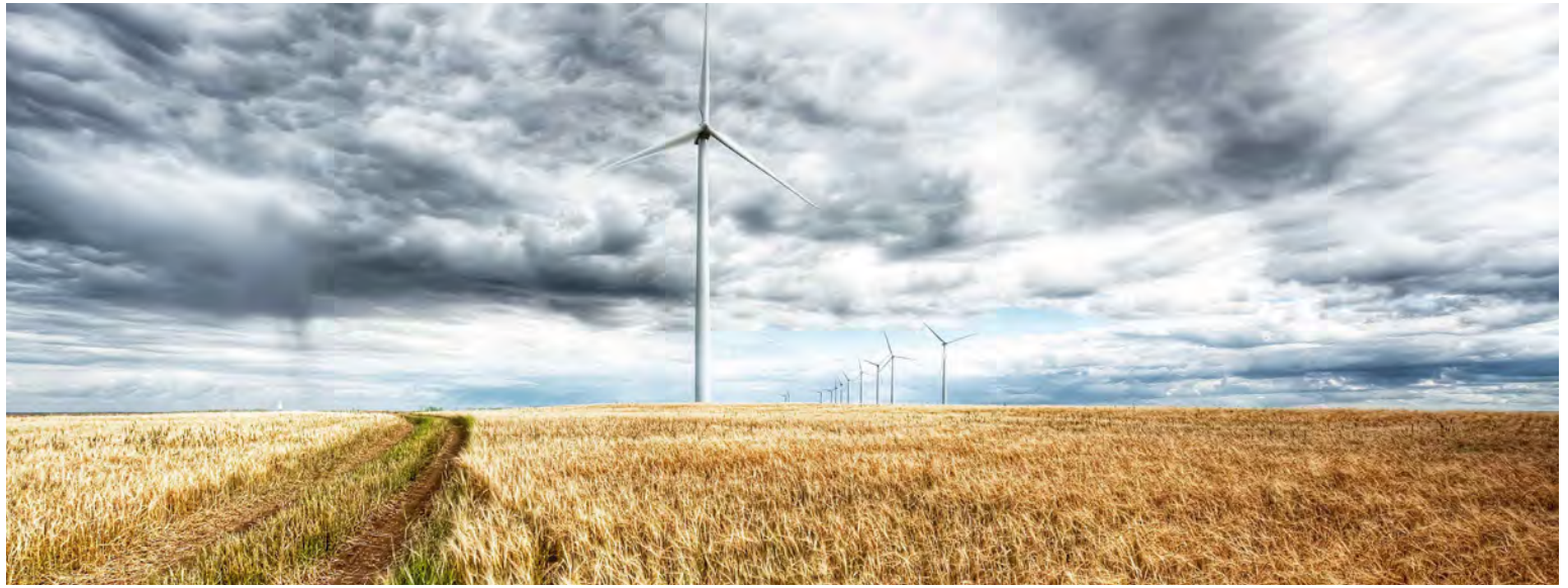
Joint venture wind project, Chin Chute, located in Taber, Alberta.
