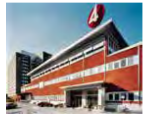
4 BREMEN During the year, TV4 extended its contract at Tegeluddsvägen. The lease, which runs from 2020, is for seven years and encompasses 13,500 square metres.
