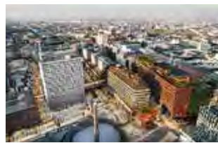
9 SERGELHUSET The transformation of Sergelhuset continued during the year. The property comprises three buildings and a total of 60,000 square metres. Tenants will move in gradually starting in autumn 2020 until the end of 2021.
