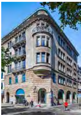
29 STYRPINNEN 15 Over the year, this property located adjacent to Kungsträdgården has been emptied and work on rebuilding and strengthening the foundations has commenced. The project encompasses 3,600 square metres and should be completed by December 2019.
