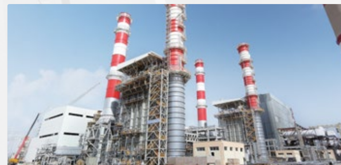
Talimarjan Combined Cycle Power Plant, Uzbekistan
