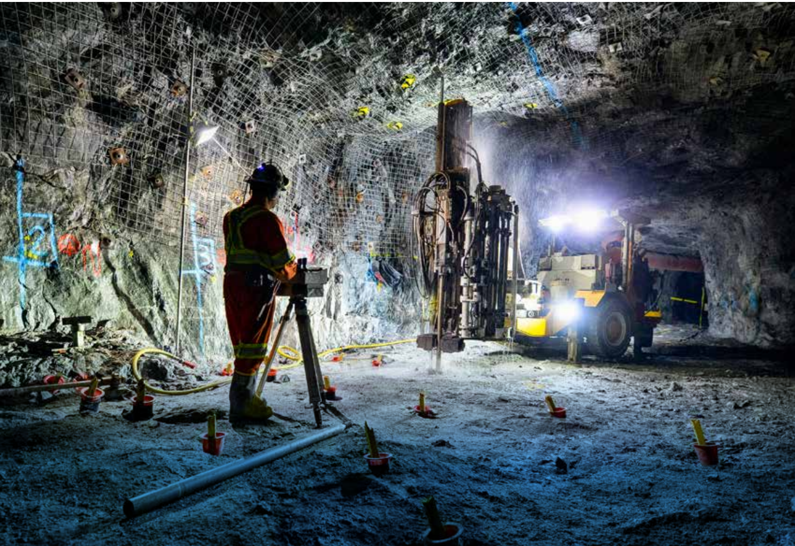
Underground at the Triangle deposit, Lamaque, Canada.
