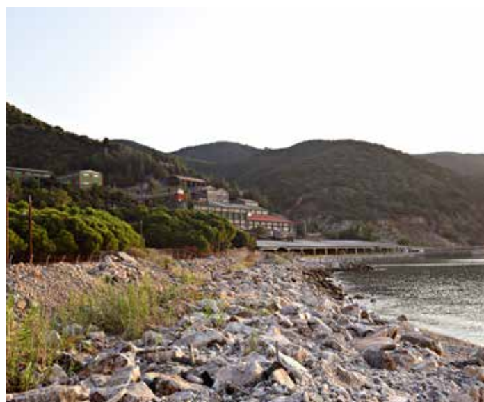
The Stratoni processing plant, Greece.
