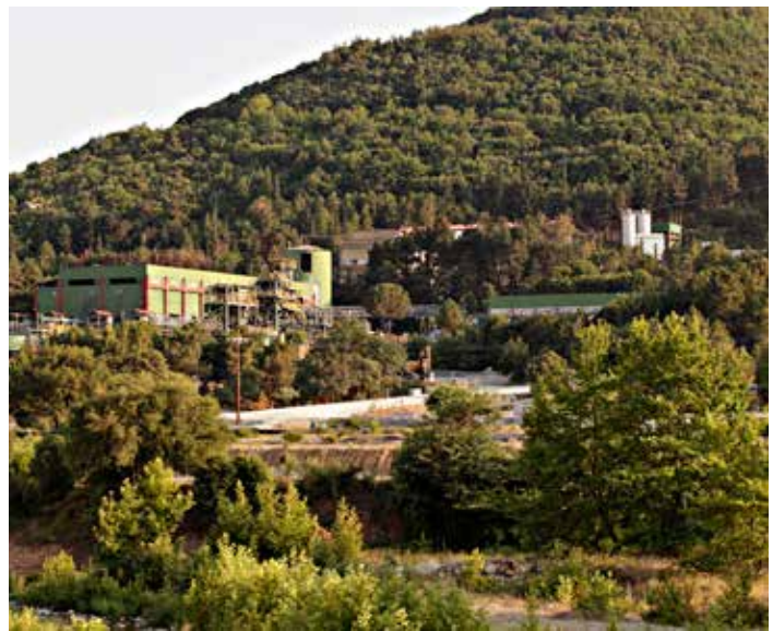
The Olympias mine and processing plant, Greece.
