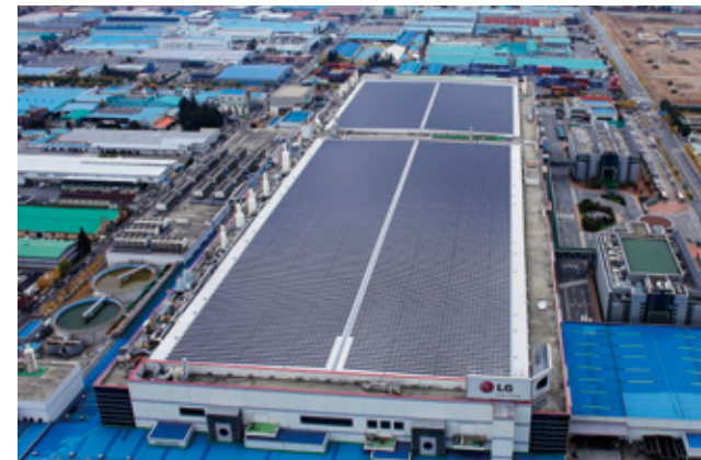
LG's PV Power Facility at Gumi Business Site
