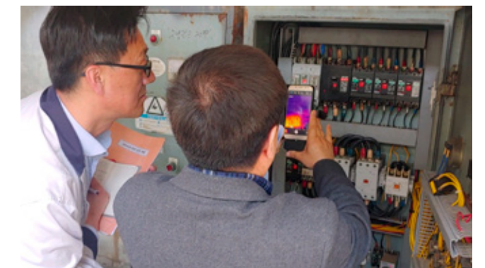
Electrical Safety Inspections to Check for Fire Risks (EPS supplier in Korea)
