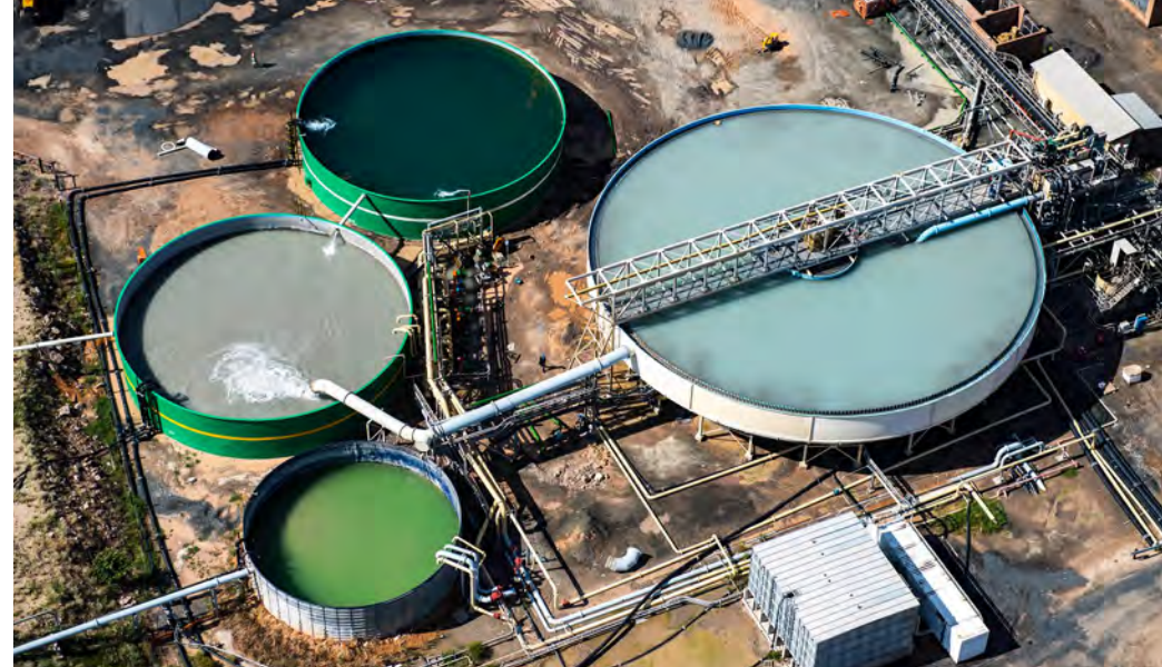
Thickener and processing water storage
