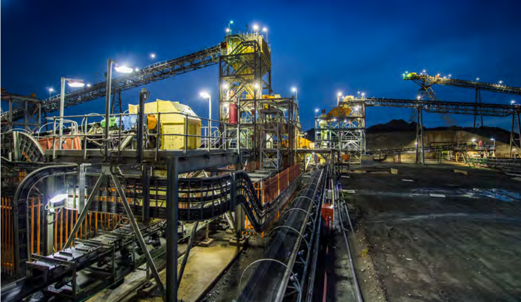
Karowe processing facility and tertiary crusher building
