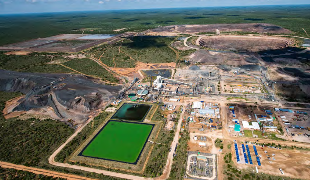
Aerial view looking west displaying water storage, processing plant and open pit
