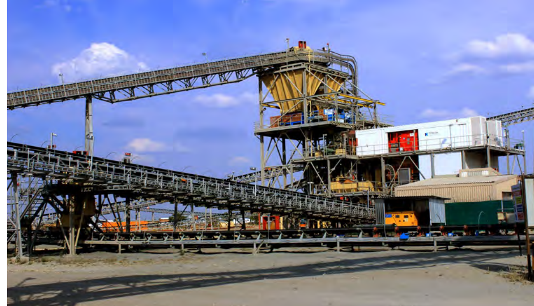
Mega Diamond Recovery (MDR) units
