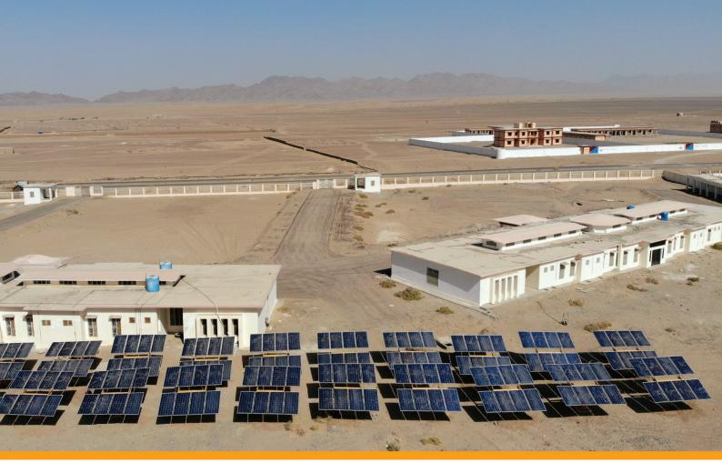
As part of the company's CSR effort to ensure consistent power supply, using renewable resource, to essential facilities in remote areas, PPL recently installed a 60 kilowatts solar system at District Headquarters Hospital and Complex in Washuk, Balochistan
