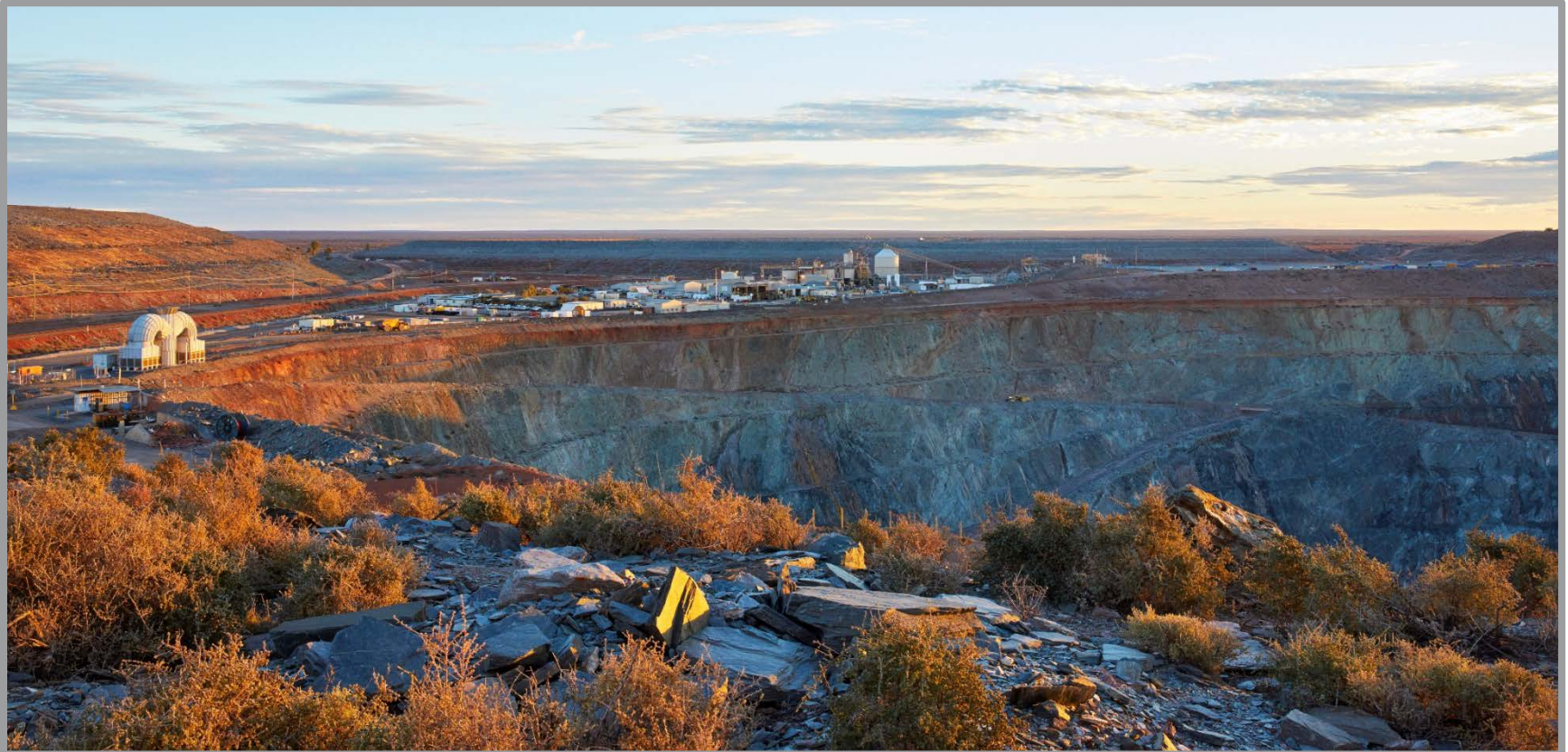
Above: Gwalia processing Plant, Leonora WA, Bulk air cooler to left, Gwalia open pit in foreground.
