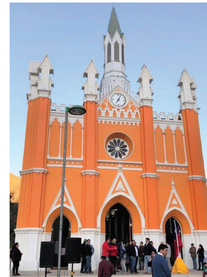
Candelaria – Church Restoration
