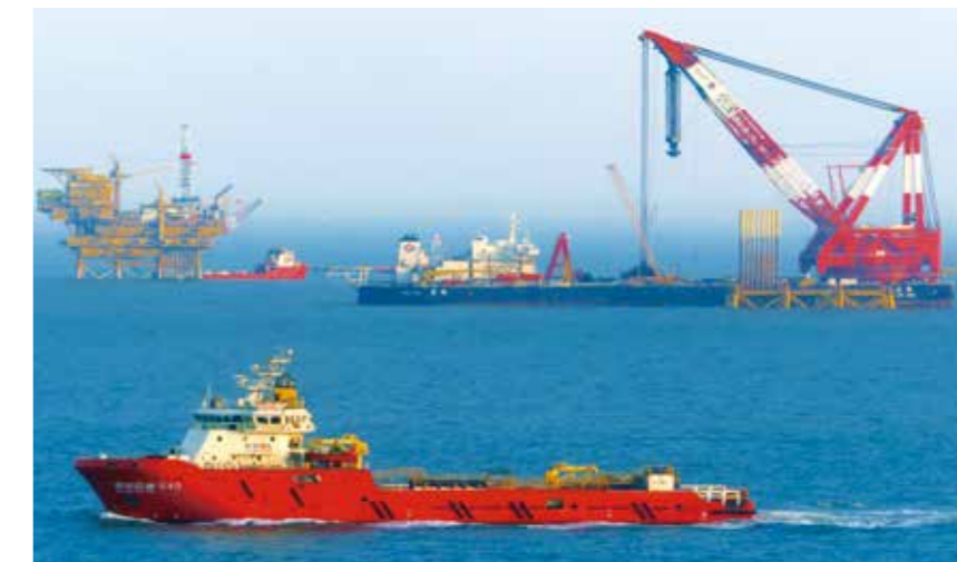
Bohai oilfield construction site
