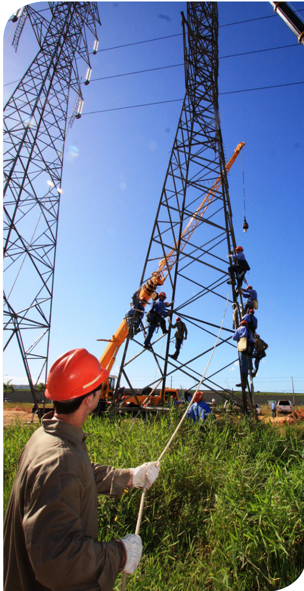
Exchange of transmission towers. Eletrobras Eletrosul collection
