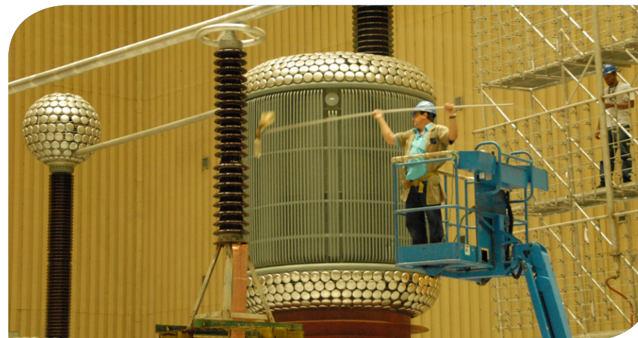
High voltage laboratory. Eletrobras Cepel / Jorge Luíz da Fonseca collection
