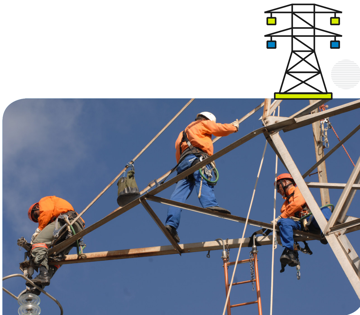
Maintenance in transmission tower. Eletrobras Chesf / Severino Silva collection
