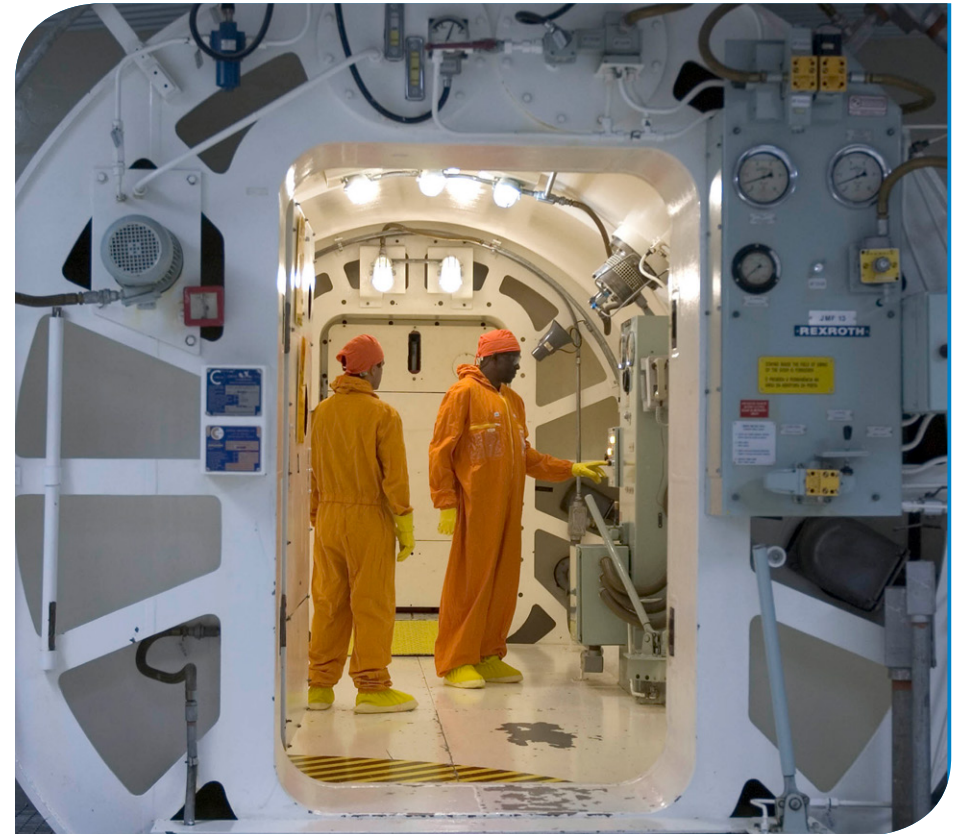
Nuclear power plant in Angra. Eletrobras Eletronuclear collection
