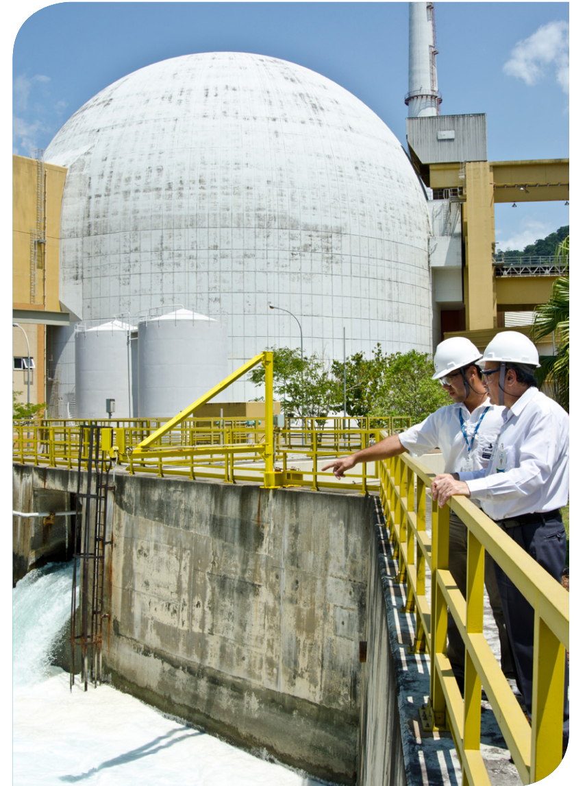
Nuclear power plant Angra 2. Eletrobras Eletronuclear collection
