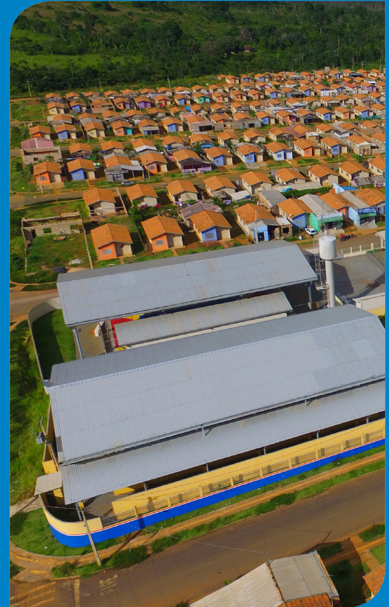
Jatobá resettlement, in Altamira. North Energy collection
