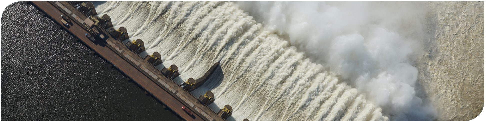
HPP Tucuruí Spillway. Eletrobras Eletronorte / Rony Ramos collection
