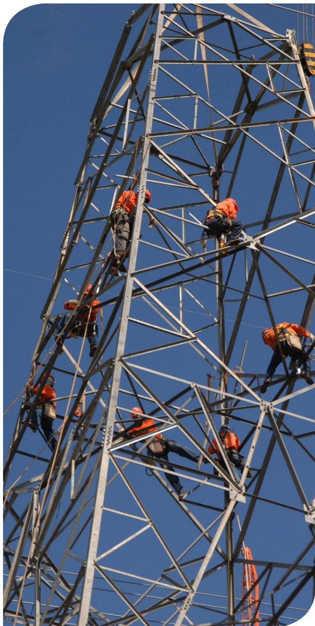
Maintenance in transmission tower. Eletrobras Chesf / Severino Silva collection
