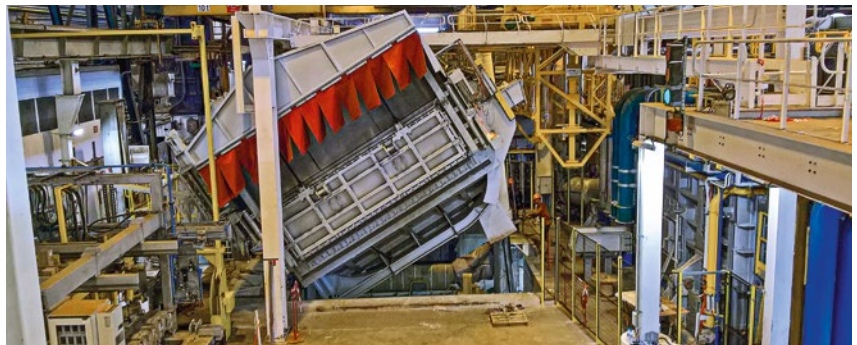
▲ Issoire’s state-of-the-art holding and casting furnaces, equipped with electromagnetic stirring for better energy efficiency.
