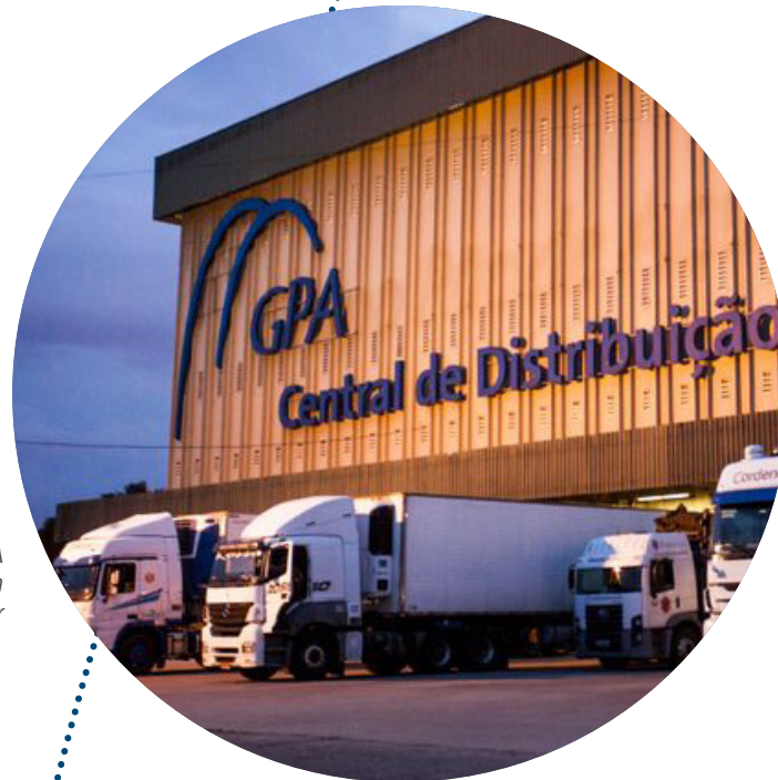
GPA Distribution Center
