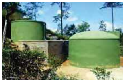
Water and Sanitation Facility
