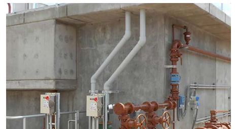
Wickenburg Ranch Water Reclamation Facility Arizona, USA
