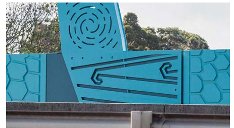
State Highway 1 Ellerslie Acoustic Barrier Auckland, New Zealand
