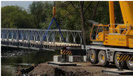
Hespeler trunk sanitary sewer line Ontario, Canada
