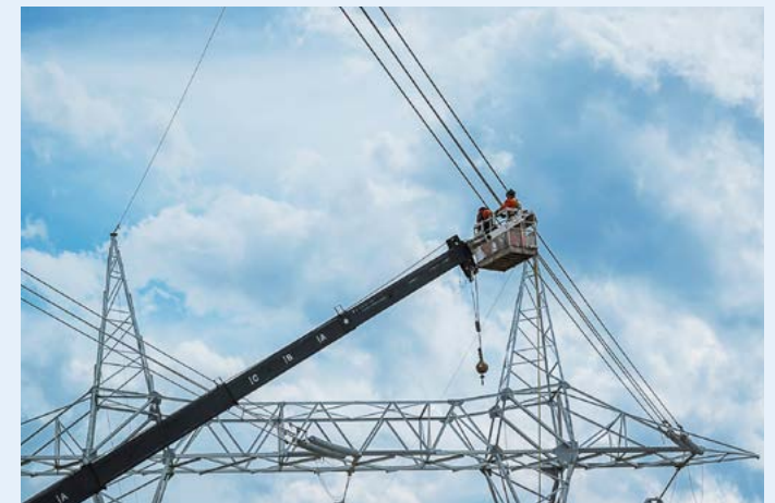
^^ Construction of the new transmission line near Highway 25.
