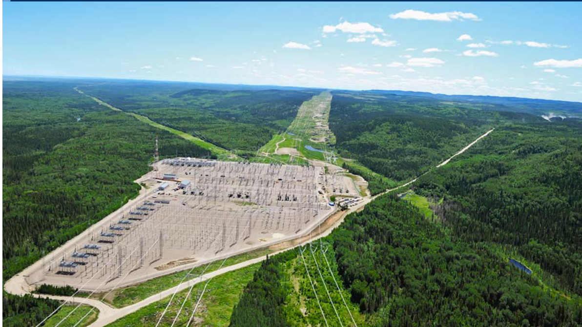
Aerial view of Chamouchouane substation
