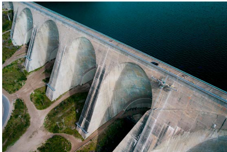
Daniel-Johnson dam, a proud symbol of Québec’s hydropower expertise.
