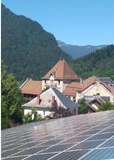
Solar panels on the RaidLight plant roof
