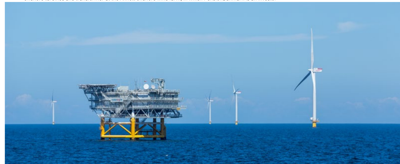
Offshore turbines and transformer at the Anholt offshore wind farm, in which PensionDanmark is an investor
