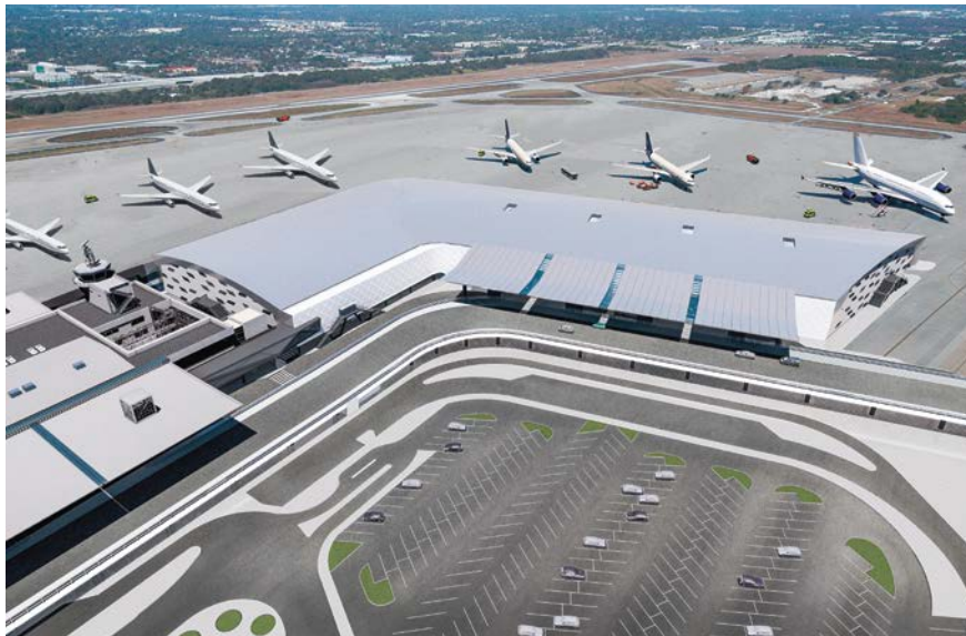
In September 2018, a symbolic ground-breaking ceremony officially marked the expansion of Thessaloniki Airport.
