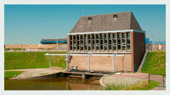
The polder pumping stations are responsible for 40% of the Scheldestromen Water Authority's energy consumption. De Dommel Water Authority has developed a new control system, which is able to handle not only high and low water levels but also weather conditions. This results in energy savings and more efficient drainage, which reduces the likelihood of flooding. It is also beneficial to fish migration, while it will counter soil salinisation and dehydration as well.
