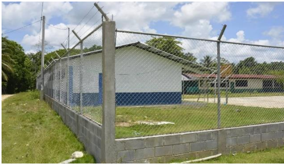
Perimeter wall in El Tamarindo school.
