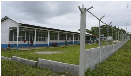
Perimeter wall in El Tucán school.
