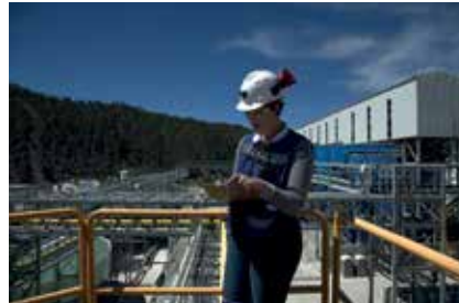
The Merrill Crowe plant at San Julián Veins.
