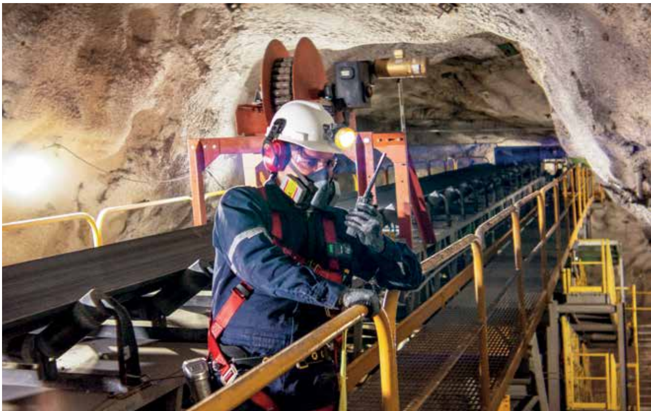
Vertical conveyor at Fresnillo.
