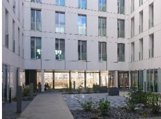
Centre de Services de Nantes - Testing
