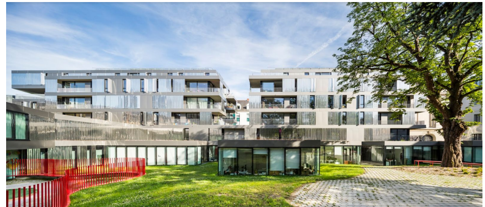
Housing complex, France - Philippe Dubus © Sergio Grazia - The project, which utilises Aperam's 304L grade with Uginox Bright Finish, won the 2018 Eiffel Trophy for Steel Architecture in the 'Living' category.
