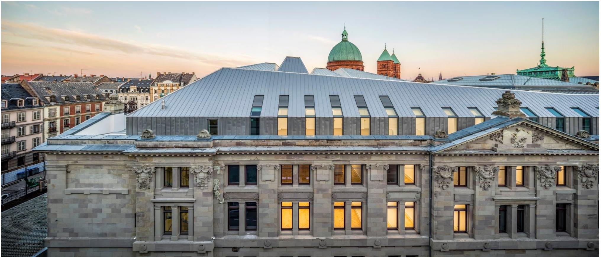
Palais de Justice (Courthouse), Strasbourg - France - Garcés.De Seta.Bonet Arquitectes & Serra-Vives-Cartagena © Adrià Goula - Executed using grade Aperam 304 with Uginox Top finish
