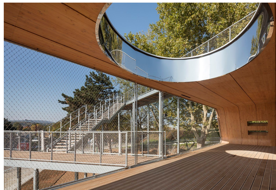
Media library, social centre and digital work space - Ropa & Associés Architectes © Luc Boegly Executed using grade Aperam 304 with Uginox Bright surface finish.
