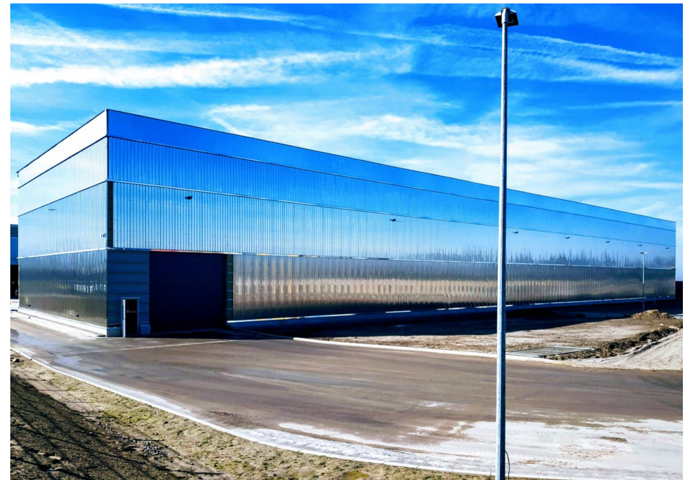
Haan: the brand-new building that will host the former Duisburg activities of S&S Germany
