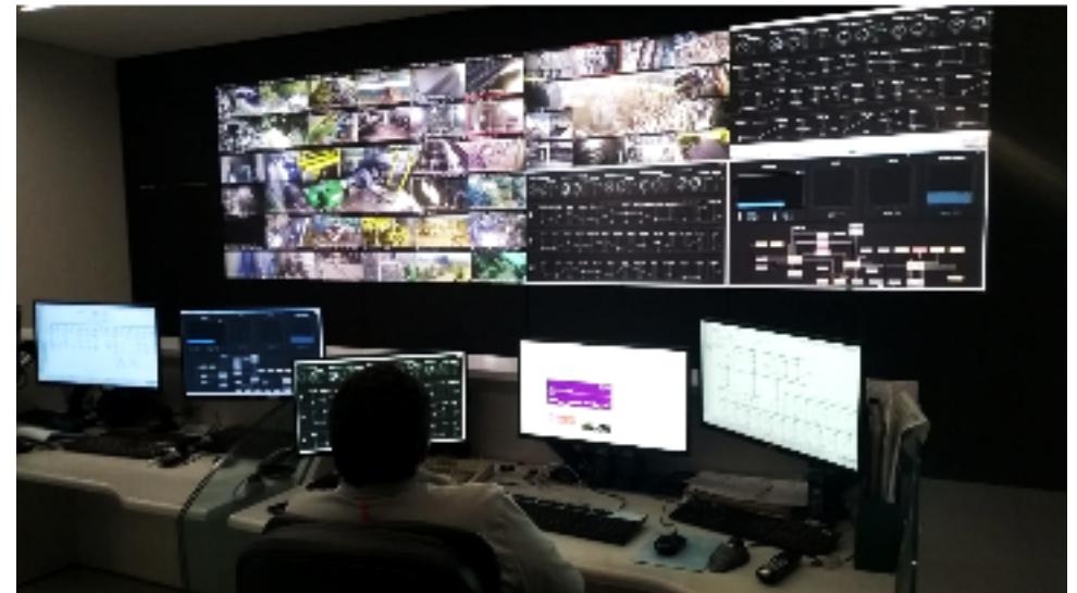
The new Integrated control center in Timóteo plant.
