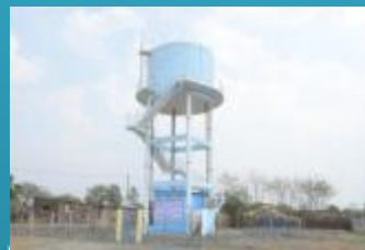
Overhead Tank, Kankund
