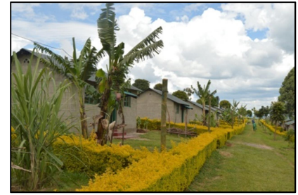
Photo1: Employee housing units in one of our estates
