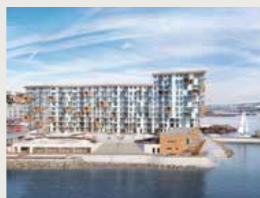
In the same area as Himmel & Hav in Tromsø Peab is building the project Skir, commercial space and 180 condominiums. Construction is in two stages, and the first 80 condominiums will be ready for occupancy in the first quarter 2021. The whole project will be completed in the fourth quarter of 2021.
