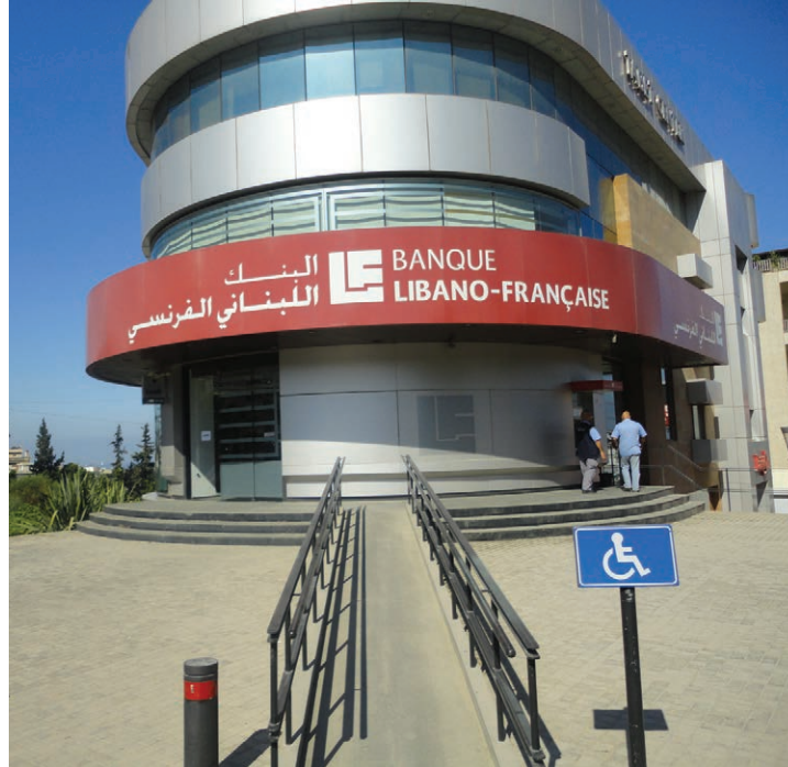
Hazmieh branch equipped with a ramp.
