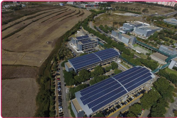
Photovoltaic solar power plant in Taguspark (Portugal)
