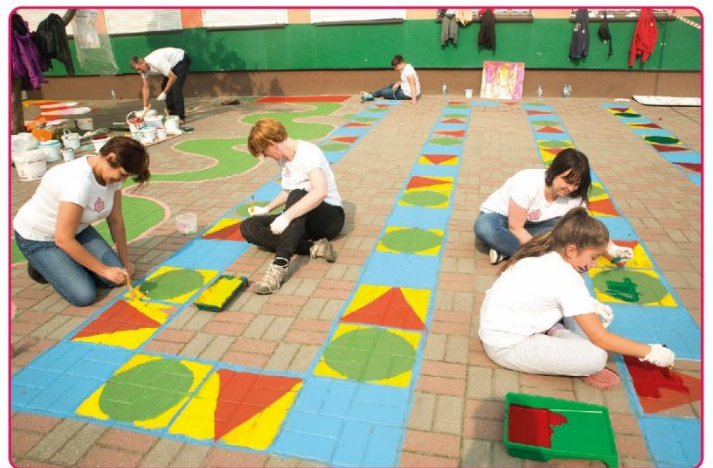
Renovation of a school playground in Czaple (Poland)
