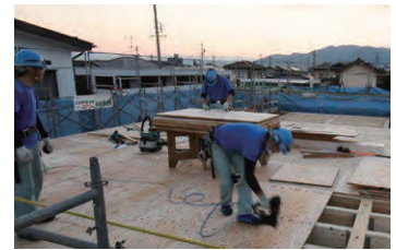
Construction using highly durable, high yield strength wall panels
