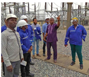
Trainees during their On-The-Job Training (OJT) at Egbin Power Station
