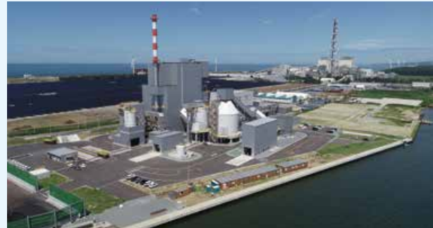
Sakata Biomass Power Plant
