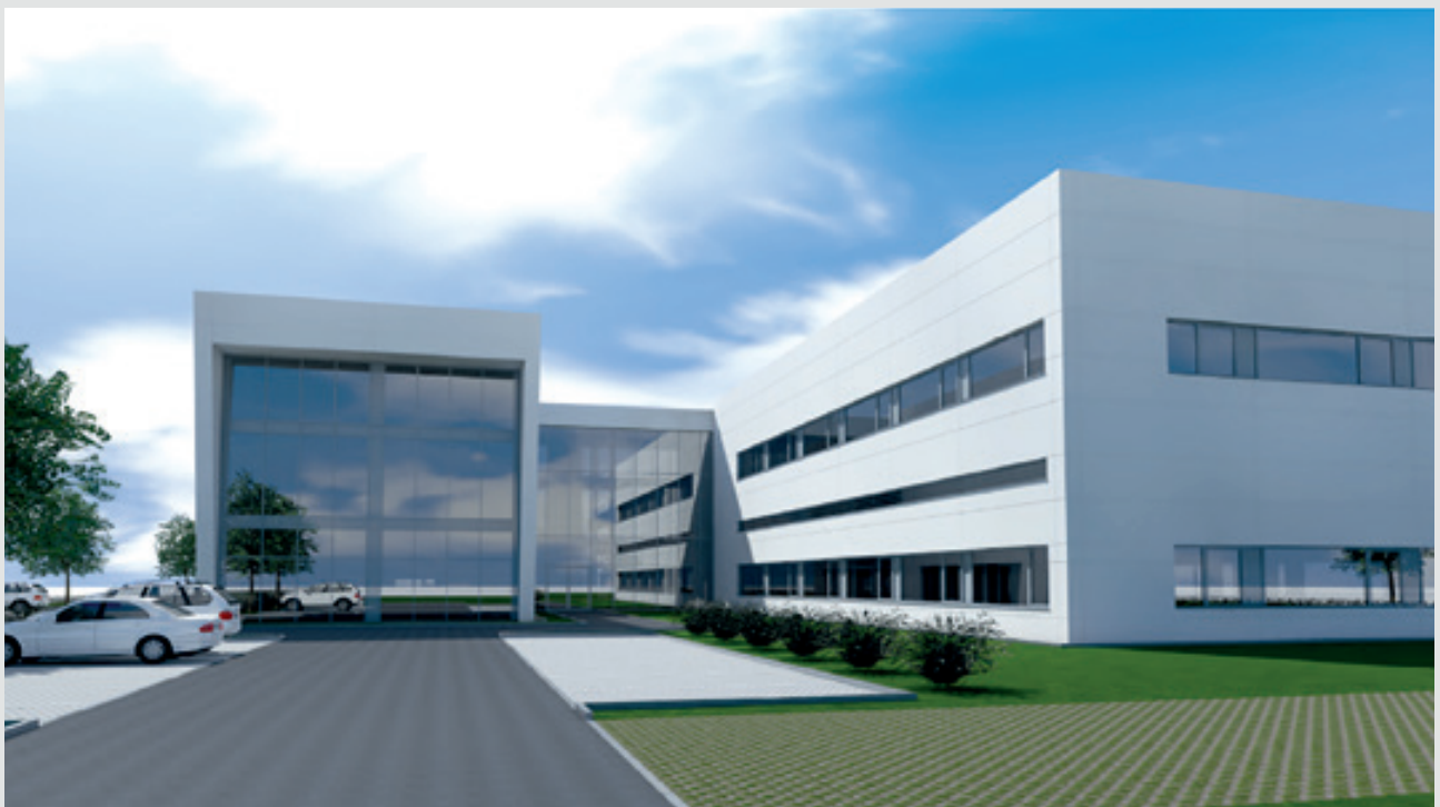
The new HEINE company building in Gilching (planning photo): On the left the 3-storey administration building, on the right the production building.
