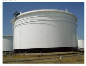
ZEFFLE applied to this tank prevents temperature rise and thus stops the contents from vaporizing
