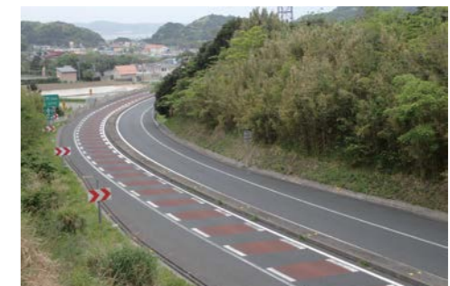
Thin-layer pavement (red pavement section)
