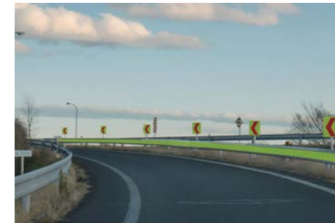
Sharp-corner guide signs and high-visibility reflective tape
