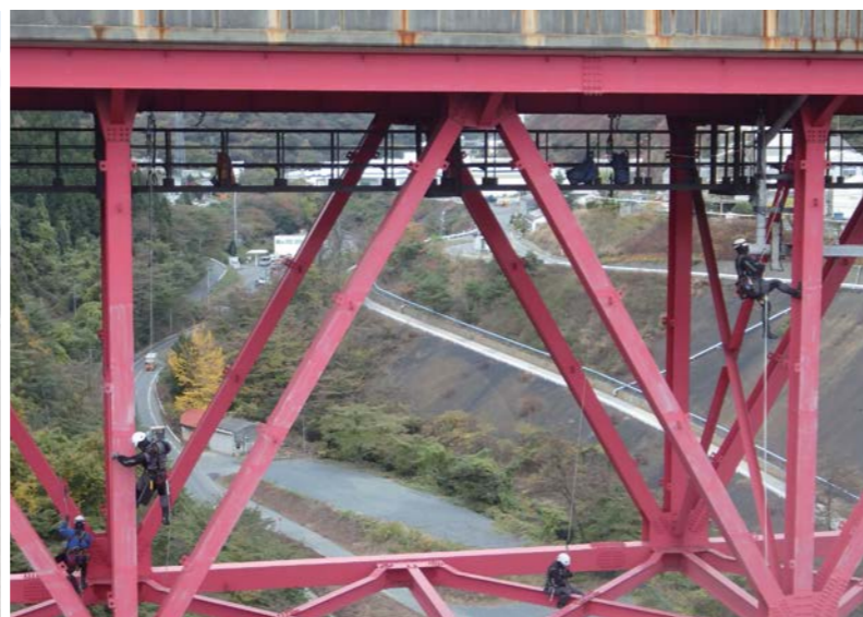
Bridge inspection via rope access
