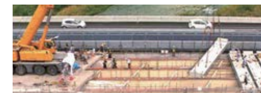
Slab replacement work
