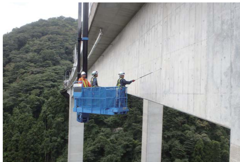
Bridge inspections (hammering test)
