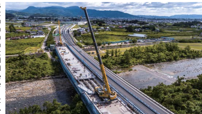
Slab replacement work
