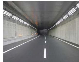
LED lighting in a tunnel
