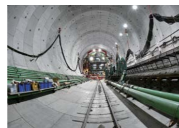
Tunnel construction using shield machine
