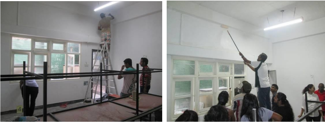
Fig 11. Factory workers lunch room renovation
