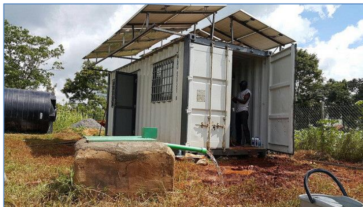
WGES WaterBox, solar irrigation system, installation in Kenya
