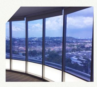
Thermal film for windows – Situated on the 8th floor with 75sqm of glasses caused of a lot of heat to be trapped inside the office. An investment in thermal transparent film to cover the glass resulted in a heat reduction of 70% and an air conditioning reduction of 3°C.
